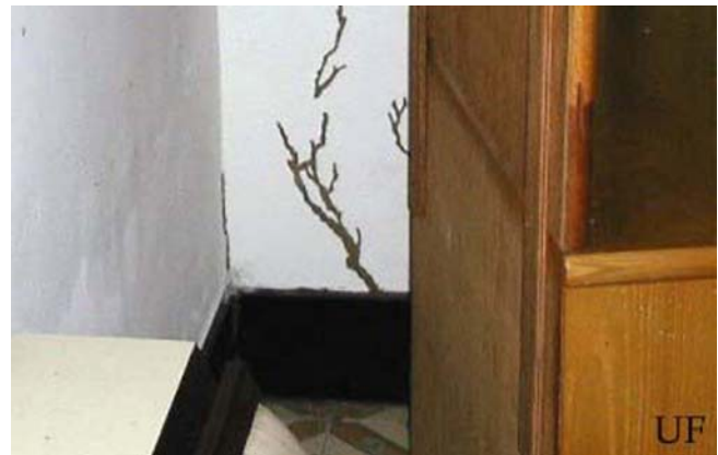
Figure 4. Soil tubes of the Formosan subterranean termite, Coptotermes formosanus Shiraki. Credits: Nan-Yao Su, University of Florida
